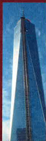
WTC In Progress January 2014
